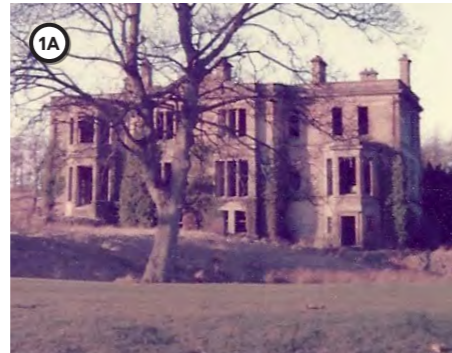
(far-left) Dougalston House (www.edicimages.co.uk) (left) The ruin of Dougalston House prior to demolition and construction of the golf course ©Elliot Simpson (www.geograph.org.uk)
