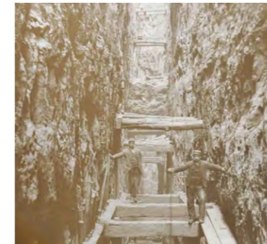
Construction of the Loch Katrine aquaduct. BBC News
